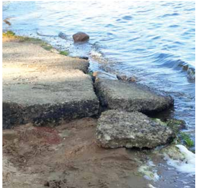
Current damaged Baptiste boat launch
